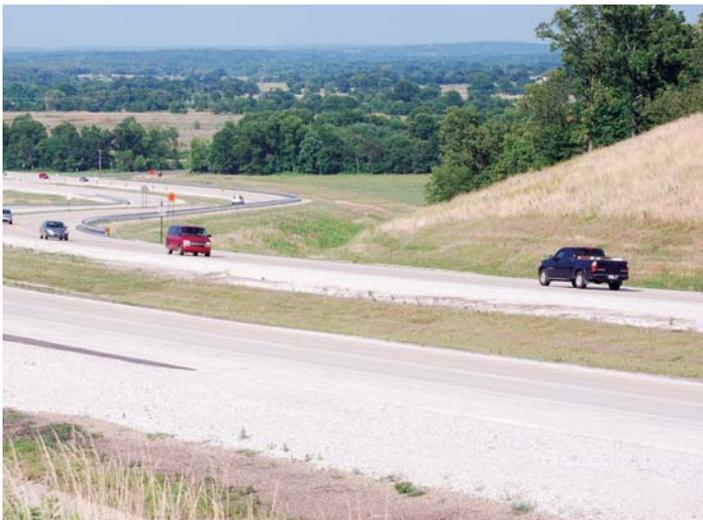
**Light Reflectance**—Concrete is naturally light-reflective, which reduces street lighting requirements (and saves energy). This enhances safety and helps reduce urban air temperature (reducing heat island effects). Darker colored paving materials cannot provide these benefits.
