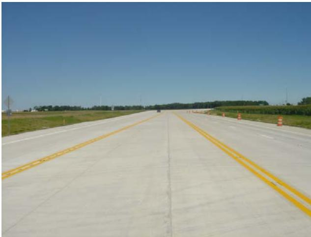
**Figure 3. Supported Edge (Tied Shoulders) of a Concrete Pavement in a Rural Setting.**
