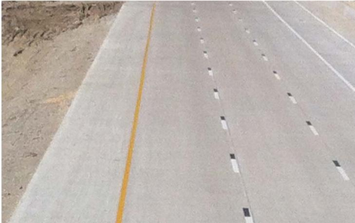
**Figure 5. Supported Edge (Inside Widened Lane) of a Concrete Pavement in an Urban Setting.**
