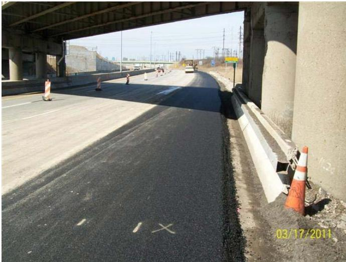
**Figure 1. Unsupported Edge (Asphalt Shoulder) of a Concrete Pavement in an Urban Setting.**
