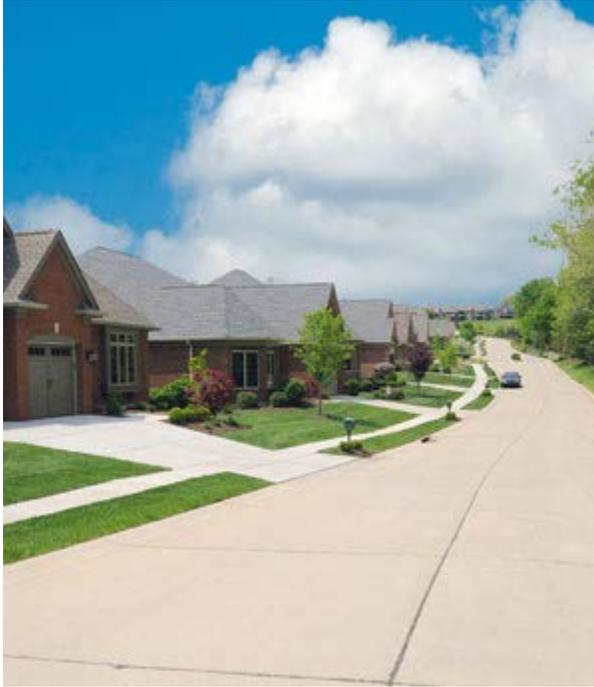
**Figure 2. Unsupported Edge (Grass Shoulder) of a Concrete Pavement in a Residential Setting.**
