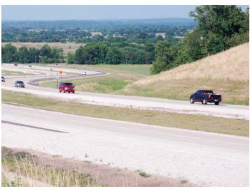
Light Reflectance—Concrete is naturally light-reflective, which reduces street lighting requirements (and saves energy). This enhances safety and helps reduce urban air temperature (reducing heat island effects). Darker colored paving materials cannot provide these benefits.
