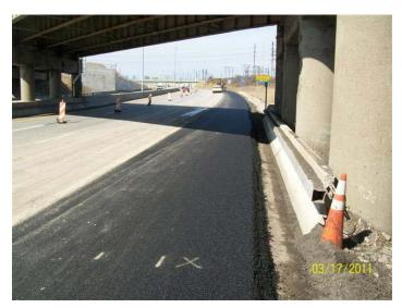
Figure 1. Unsupported Edge (Asphalt Shoulder) of a Concrete Pavement in an Urban Setting.
