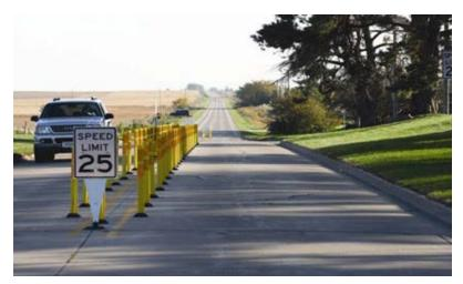
Figure 4. Supported Edge (Curb & Gutter) of a Concrete Pavement in a Rural Setting.
