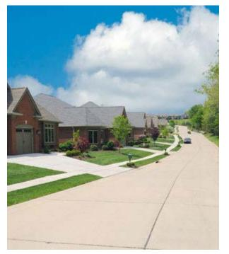
Figure 2. Unsupported Edge (Grass Shoulder) of a Concrete Pavement in a Residential Setting.
