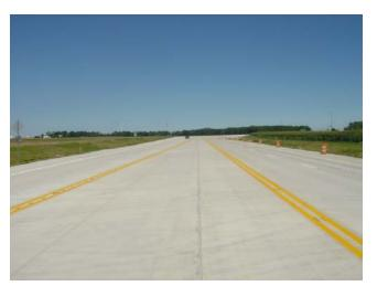
Figure 3. Supported Edge (Tied Shoulders) of a Concrete Pavement in a Rural Setting.
